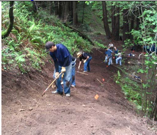
Volunteers building a new park trail
